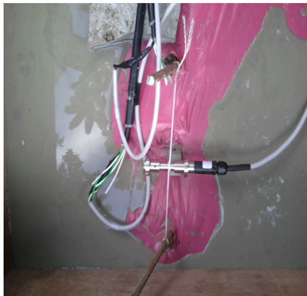
FIGURE 2. PLACING OF VIBRATING WIRE STRAIN GAGE IN PAVEMENT TEST STRETCH
